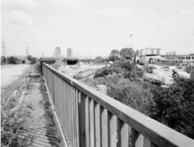
The Northern Outfall Sewer, 2003
