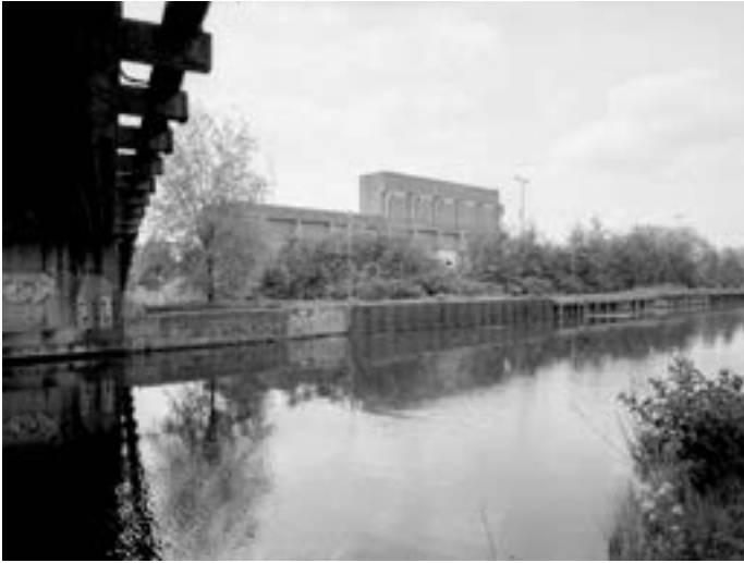
The remains of Lea Bridge Power Station, 2003
